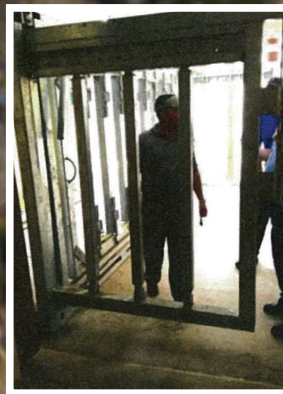
Meyer De Kock, Manager, inspecting the TAMER™ manual slide door with adjustable vertical pickets.
